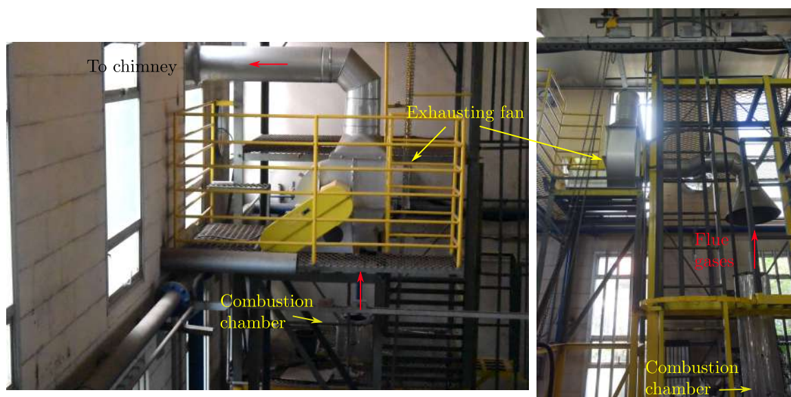
Figure 3.9 – Flue gas extraction system.
