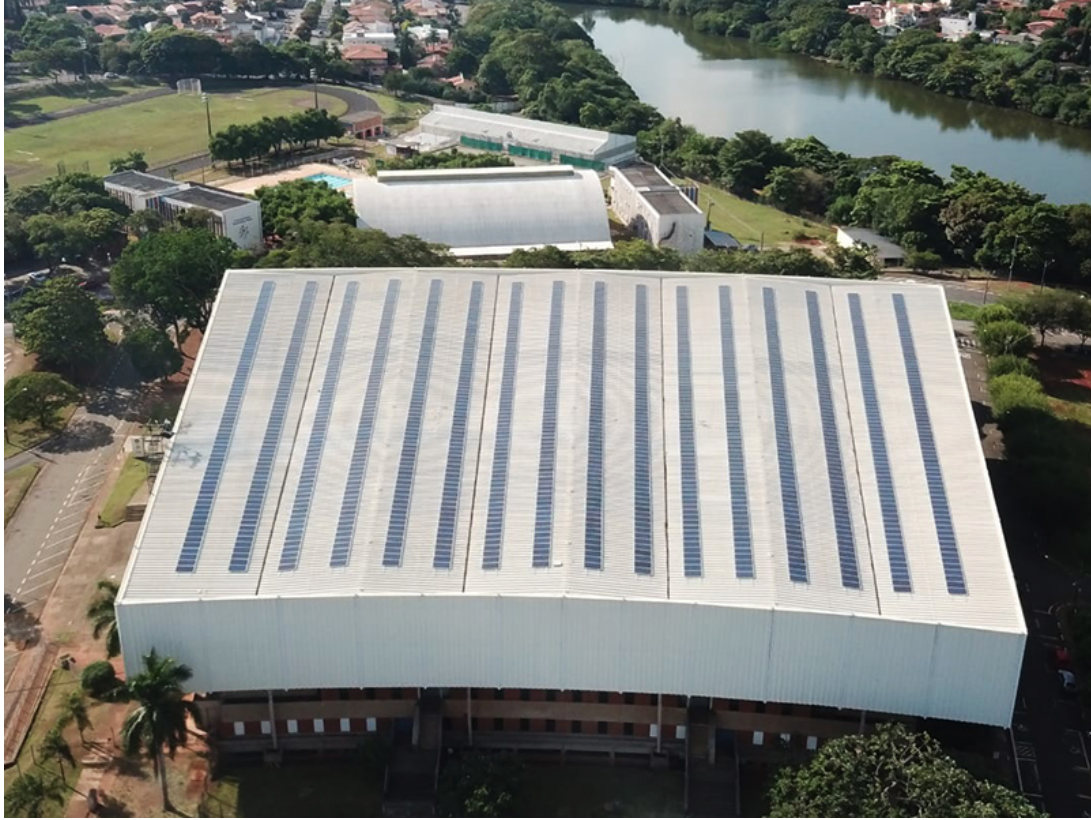
Figure 5.6 – PV installation at the Unicamp Gymnasium [33].
