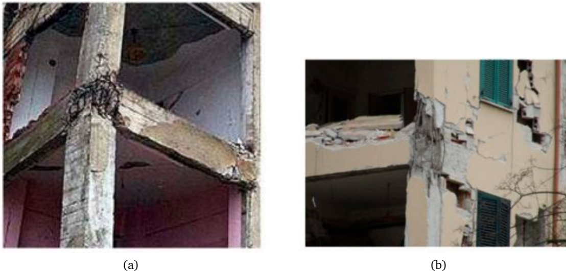
Figure 1.1 – Failure in corner BCJ caused by earthquakes: a) Earthquake Izmir in Turkey 1999, b) Earthquake Abruzzo in Italy 2009.
