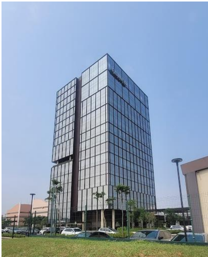
Figure 39 - Galleria Smart corporative centre (Smart Building)
