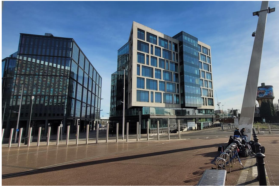
Figure 6 - Class A buildings in Cardiff Enterprise Zone
