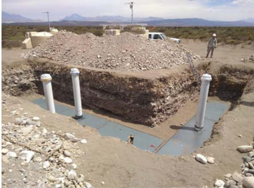
Figure 4.5: Installation of an Underground Muon Detector (**UMD**) unit at a depth of 2.3 m. The three modules are arranged in an "L" shape, collectively covering an area of 30 m<sup>2</sup>. Each module is composed of 64 scintillator bars with embedded wavelength-shifting fibres that guide the produced light to 64 **SiPMs**. The equipment is housed in a **PVC** enclosure, where a **PVC** tube is connected for installation and easy maintenance.
