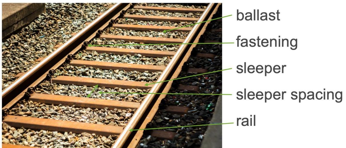
Figure 2: Main components of the rail track superstructure - (CARLVIK, 2020).
