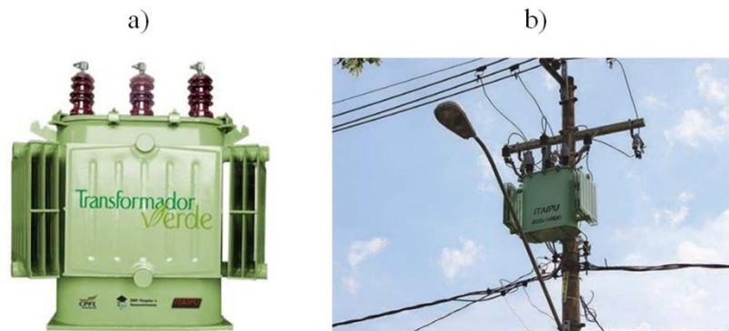
Figure 10: A. CPFL green transformer (CPFL, 2017); b. Itaipu distribution transformer 13.8 kV voltage level (Vasconcellos, Mak, & Jr, 2014).
