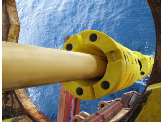
Figure 3.11: Example of subsea buoy module for oil pipeline support (image extracted from Flotation Technologies ® website at the url http://www.flotec.com/products/buckle-migration-buoyancy-modules , in 18th September, 2013).
