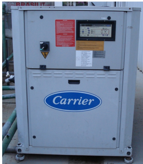
Figure 3.1. Equipment used to control the temperature of the bath during the restart flow tests and during the cleaning of the pipeline (Luthi, 2013).
