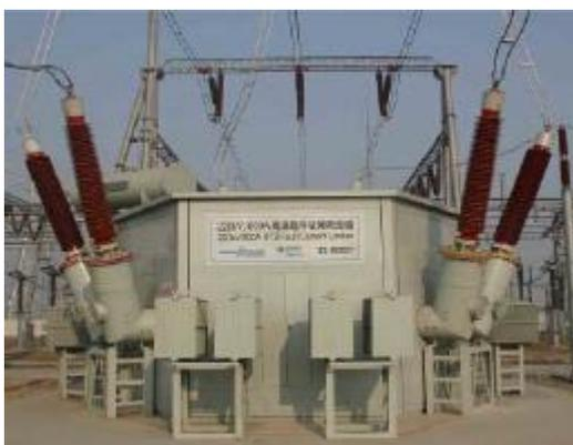
**Figura 3.23: LCESENS da Innopower de 220kV/300MVA [40]**
