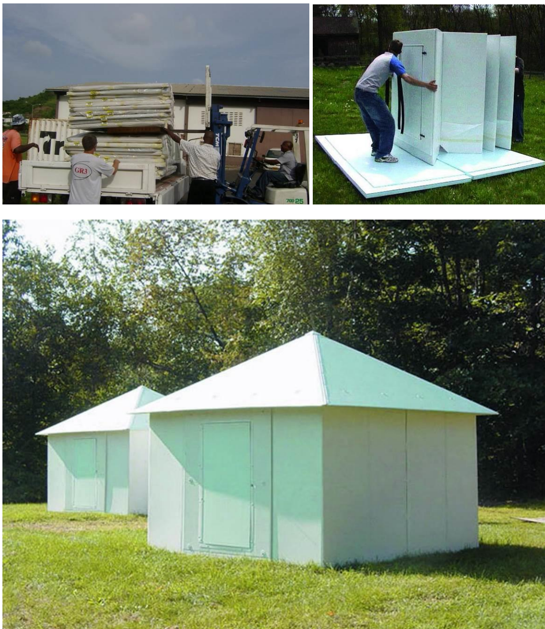
Figura 4.2.2.2 Transporte e montagem do Global Village Shelter
