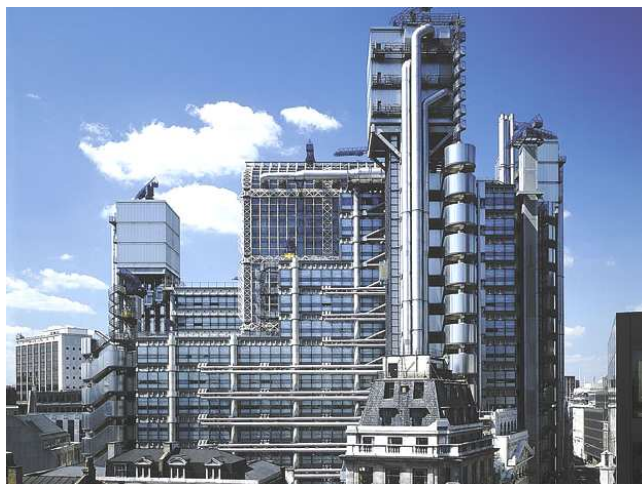
Figura 3.32 - Loyds Bank - Arquiteto Richard Rogers - Londres (1977-1984) (Fonte: < http://www.richardrogers.co.uk/work/selected_works/lloyd_s_of_london >)
