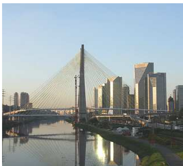
Figura 3.50 - Ponte Octavio Frias de Oliveira (Ponte Estaiada) - São Paulo (SP) - 2008 (Fonte: < http://farm4.static.flickr.com/3226/2457913237_6997f5630f.jpg?v=0 >)
