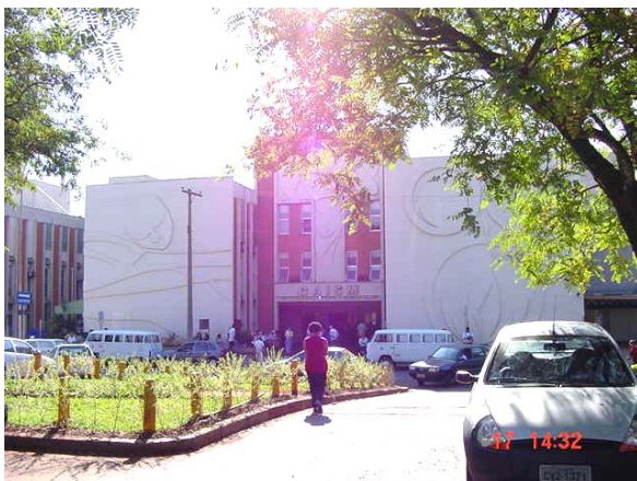
Fachada principal do CAISM/DTG/Unicamp
