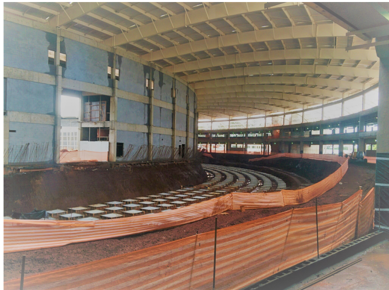
Figure 1.1: Stage of the construction of the Sirius facilities - large group of piles.
